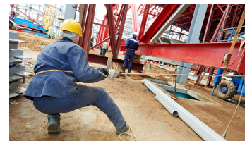
Safety Awareness Monitoring
