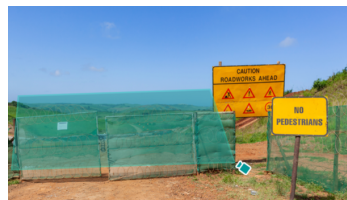
Perimeter Intrusion Detection
